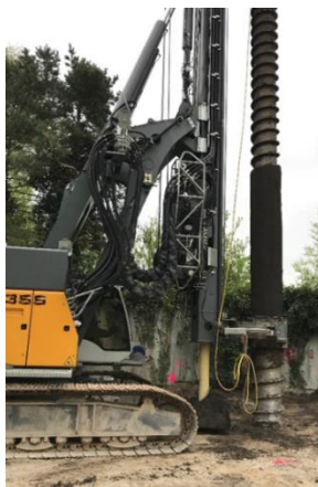
Figure 1: The optical fiber cable is fitted into the pile mould, before the concrete is poured in.
